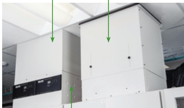
Example of both Passive and Active Chimney Systems
