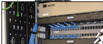
Lacing Panel shown in enclosure
