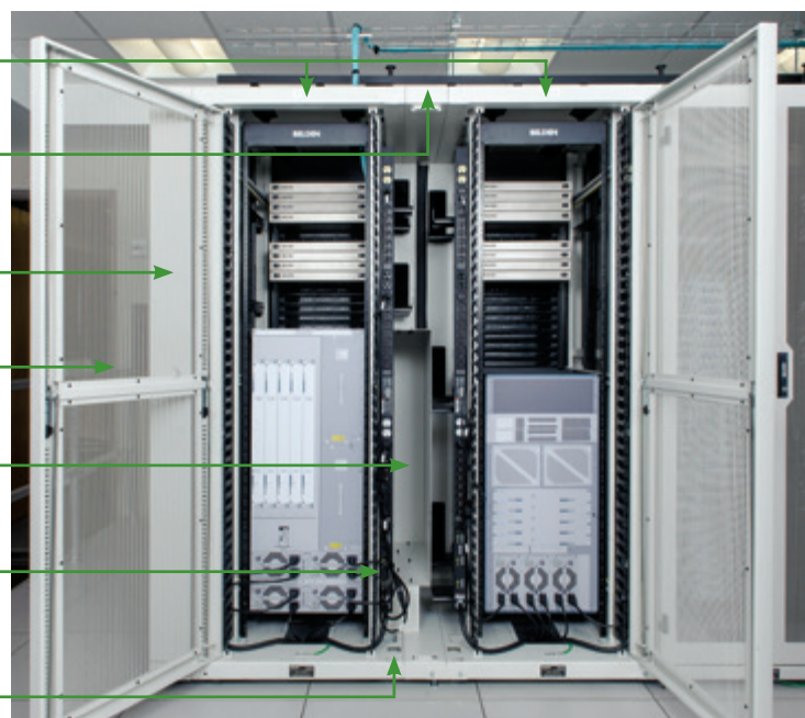
Ganged XN frames with end-of-row 6" extension and between enclosure 6" extension (rear view)
